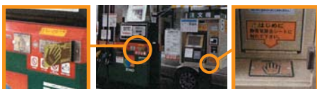
Measuring instruments and POS machines fitted with static electricity removal sheets
