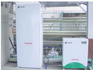
LPG-reforming type stationary fuel cell system
