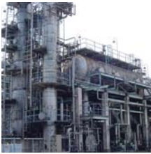
Sulfur recovery and tail gas treating unit
