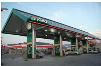
A service station with photovoltaic power generation panels installed
