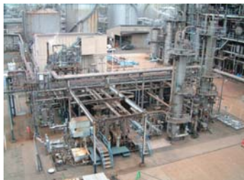
Liquefied carbon dioxide units Carbon dioxide gas released from the refinery is collected and purified, and liquefied carbon dioxide is produced.
