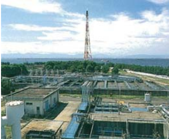
Wastewater treatment facilities
