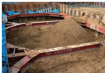
Backfilling works at the former Funakawa Oil Refinery
